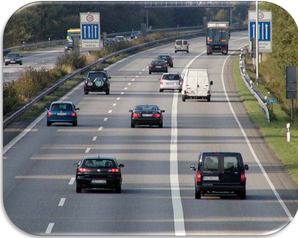
Figure 5. Photo. Temporary Shoulder Use—Germany (13) .
