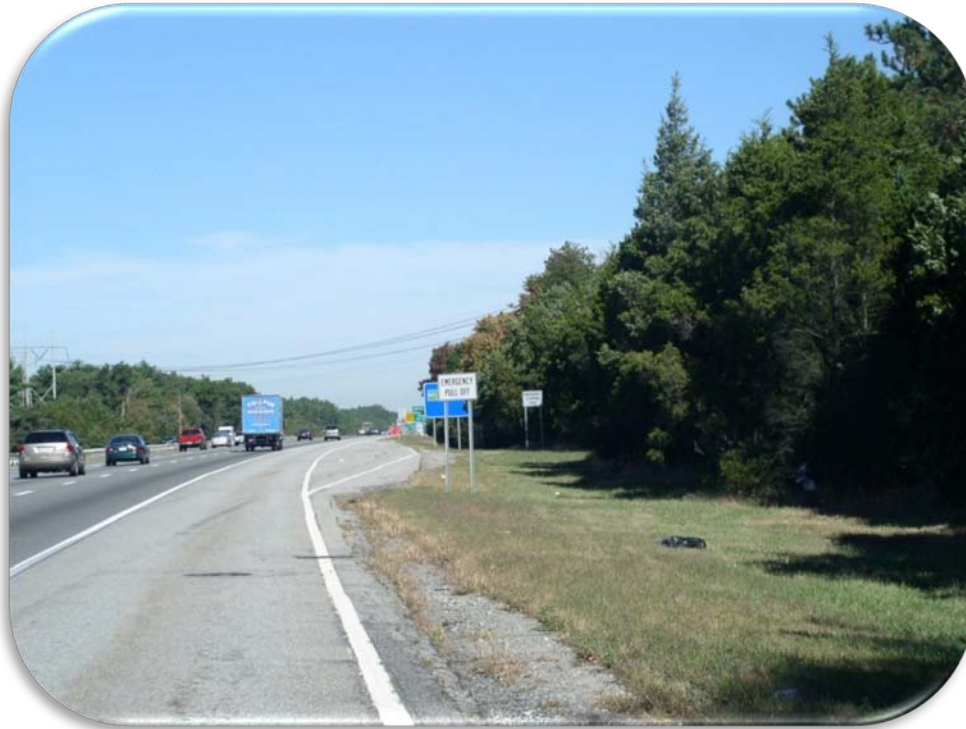
Figure 46. Photo. Breakdown Shoulder Use on I-93—Massachusetts. (23)
