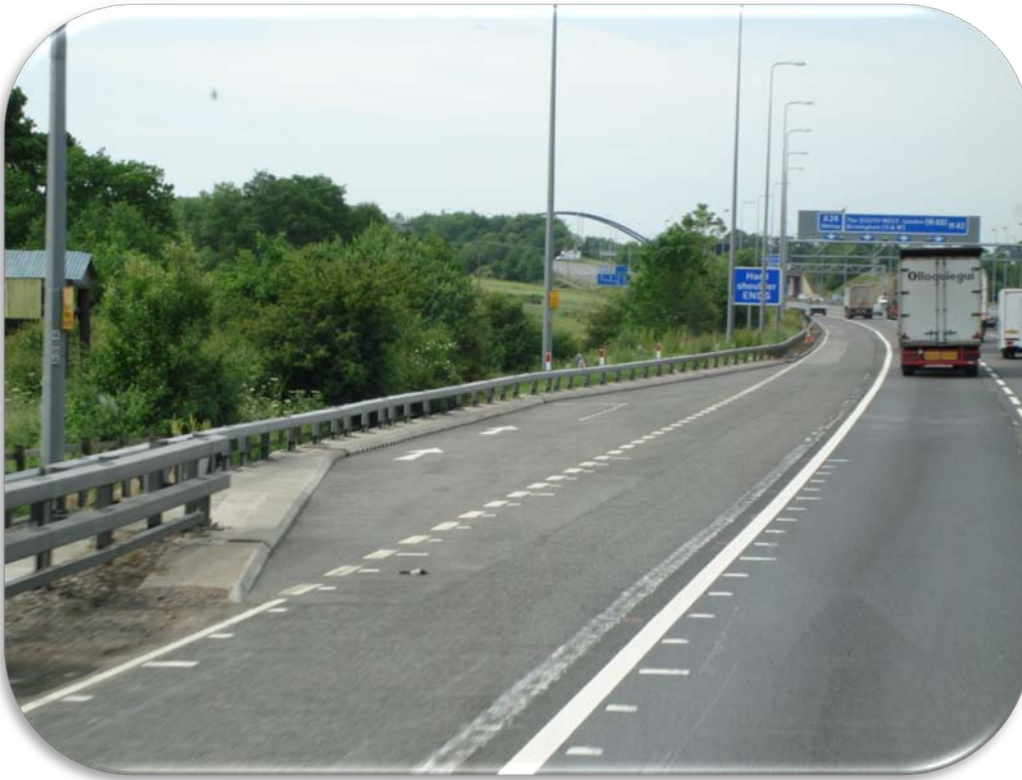
Figure 6. Photo. Shoulder Use with Emergency Refuge Area—Great Britain. (1)
