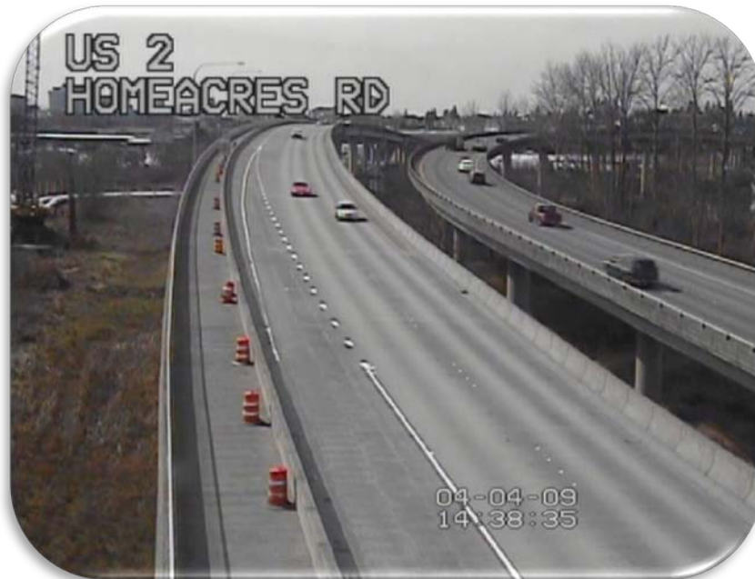
Figure 47. Photo. US 2 Shoulder Use—Everett, Washington. (55)
